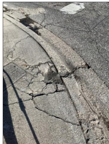
Cracked sidewalk at the southwest corner of the Silver Star Road intersection. Doesn't appear to be ADA compliant. (Source: HDR)
