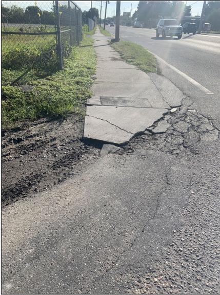
*Sidewalk cracking at Regent Ave. Not ADA compliant. (Source: HDR)*
