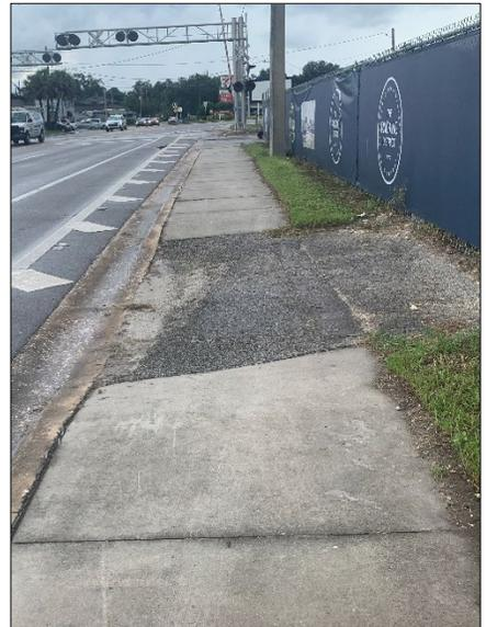
Sidewalk on the east side of Princeton Street just south of the at-grade rail crossing at a driveway leading to Packing District. The slope of the driveway doesn't appear to be ADA compliant. (Source: HDR)
