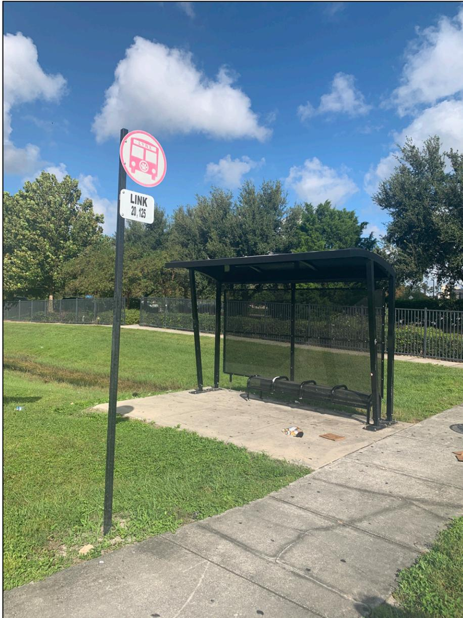
*Bus stop on the north side of Princeton Street in front of Walmart. The stop has a shaded bench and concrete slab and appears to be in good condition. (Source: HDR)*
