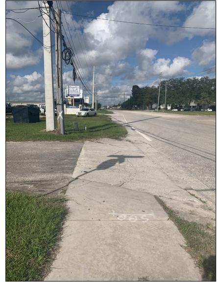
*Sidewalk at the Citgo gas station driveway. The slope of the driveway doesn't appear to be ADA compliant. A sidewalk gap can be observed beyond the driveway. (Source: HDR)*
